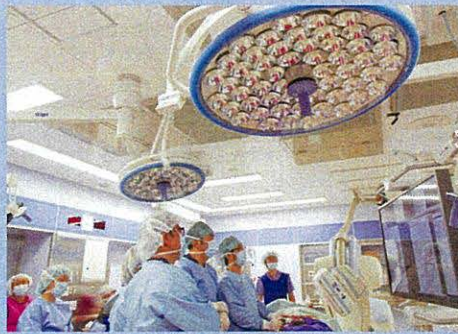
Hybrid operating room
